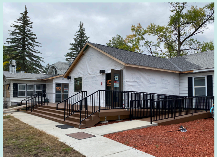
The $4.3 million construction continues at St. Cloud Youth Shelter.
